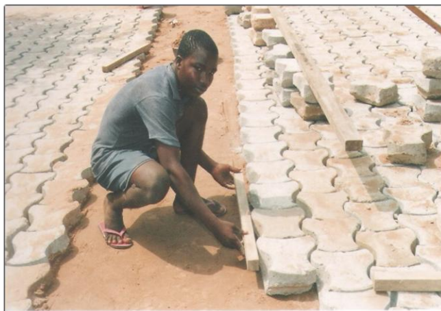
Figure 8. Work in implementation (laying pavers on the downstream slope) (2003)
