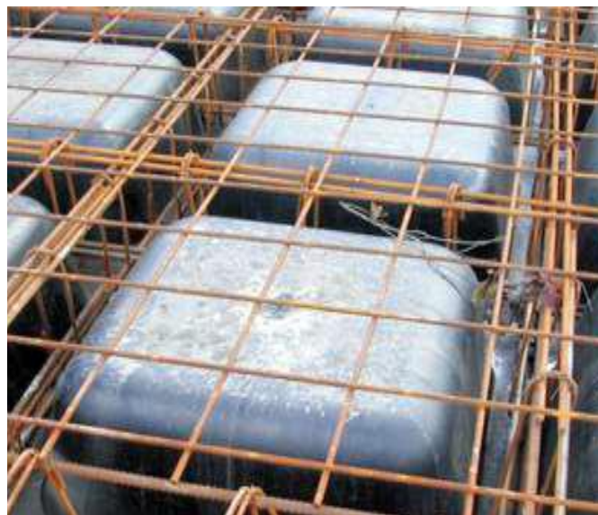
Figure 8. Waffle slab steel placing
